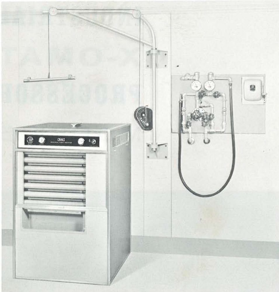
TYPICAL INSTALLATION OF KODAK INDUSTRIAL X-OMAT PROCESSOR, MODEL B
